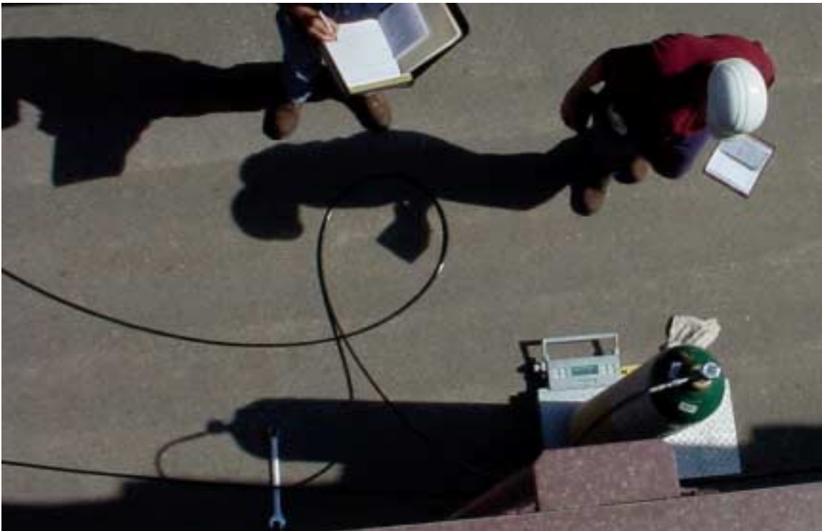
Figure 5. ECO 2 FUME® cylinder and scale during addition
